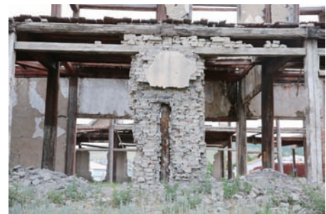
Insertion of a column into the wall
