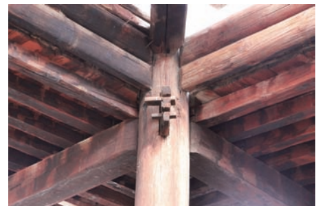
Rake-joining of columns
