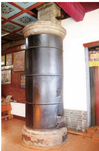
kiln stove of Sandui dugan
