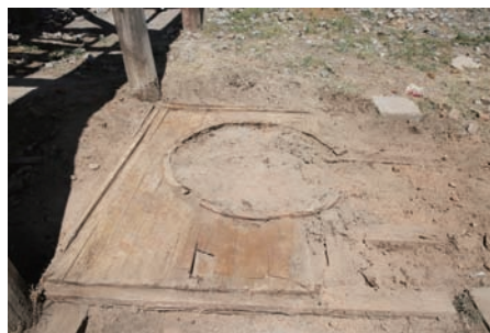
Floor structure of the western center
