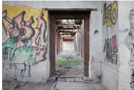
Internal door of the western side room
