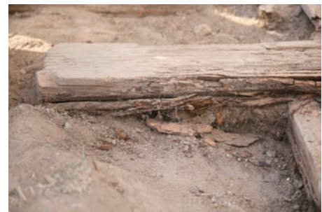
Details of the eastern floor materials
