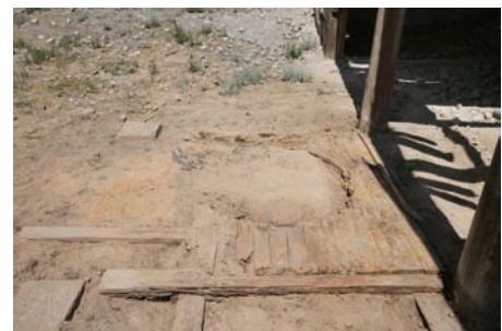
Floor structure of the eastern center
