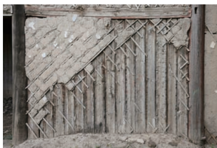
Bracing of the inner wall
