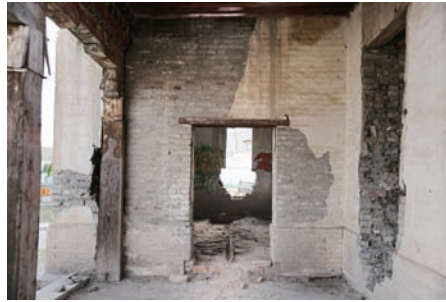
Door to the western side at the front
