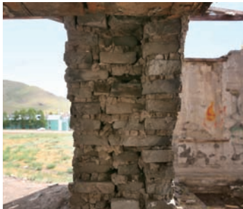
Masonry wall section
