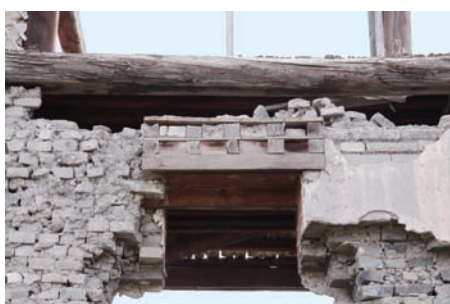
Top of the window at the elevation on the east side
