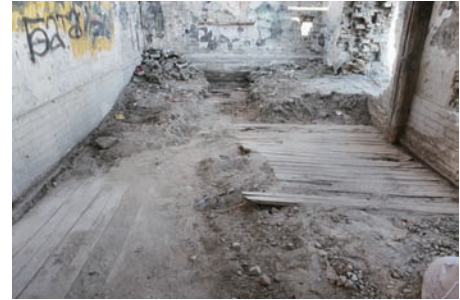
Wooden floor of the eastern side room at the front
