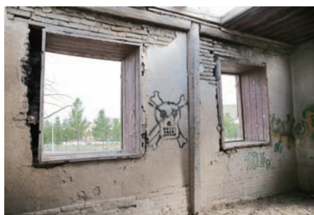
Inside the window on the west side
