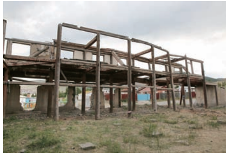
Internal column of Tsogchin Dugan
