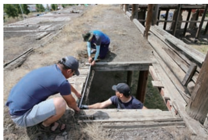
Survey of the frame structure of the upper part
