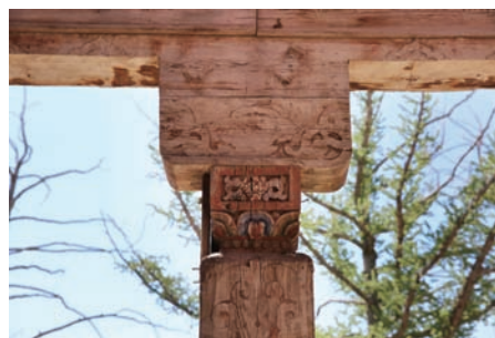
Pattern and paintwork on top of columns at Tsogchin Dugan (1)
