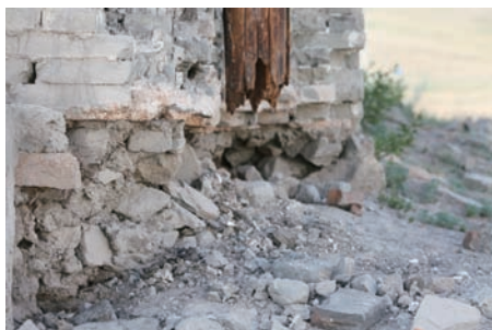
Piling rubble stones for the stylobate
