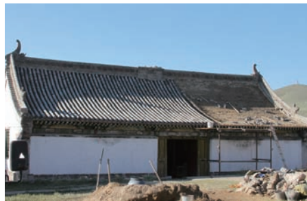
Roof restoration work in 2012
