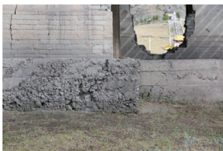
Stylobate finished with concrete (1)
