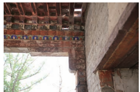
Pattern and paintwork on top of columns at Tsogchin Dugan (2)
