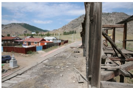
West side of the roof of Tsogchin Dugan
