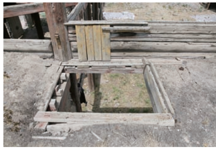
Entrance opening of the upper and lower stories Log frames and floorboards on the upper story
