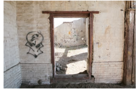
Door to the eastern side room at the front
