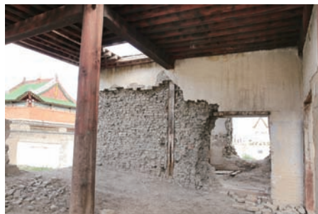
Interior of the masonry wall
