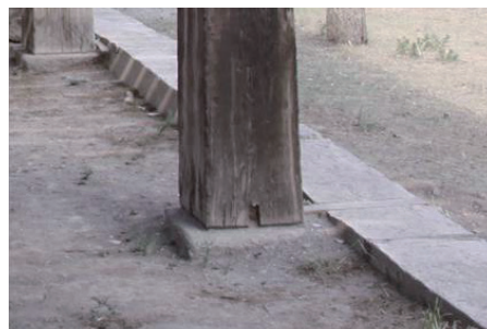
Square foundation stone at the front
