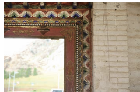
Details of the southern door's design
