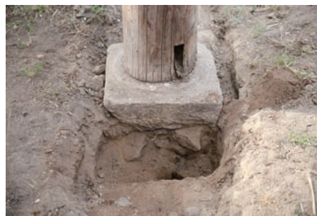
Square-shaped foundation stone for round column and rubble stone
