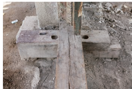
Doorpost and supporting wood of the southern door
