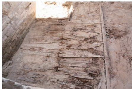
Wooden floor details of the western side room
