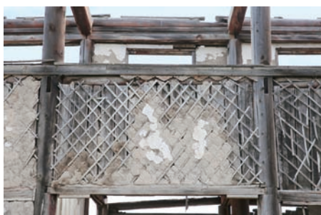
Bracing and mud-plastered wall of the inner wall
