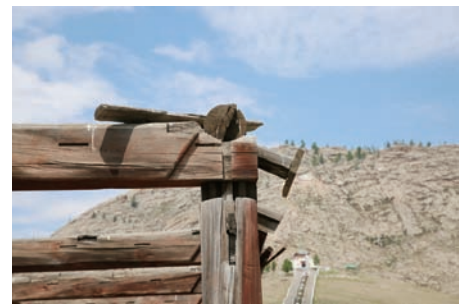
Crossbeam and girder joining of the top part of the columns
