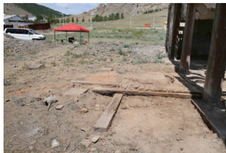
Main prop under the floorboards and common joist of the eastern floor
