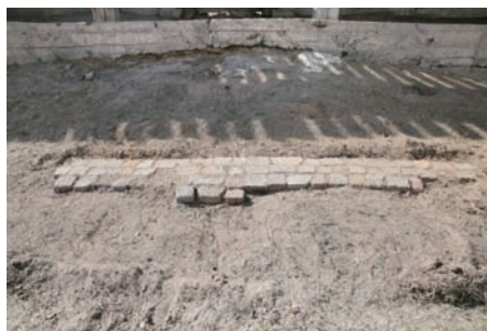
Front-side ground finishing
