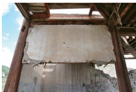
Finishing of the inner wall with plaster
