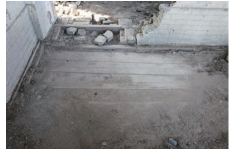
Traces of an internal door of the eastern side room
