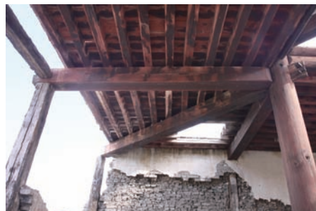
Joining of the beam between the plain columns of the lower story
