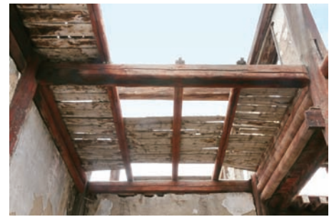
Entrance opening of the upper and lower stories Log frames and floorboards on the upper story
