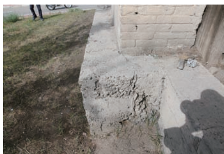
Stylobate finished with concrete (2)
